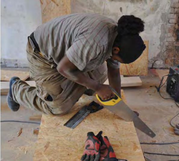
Student Albeda-collega reneveert woning
